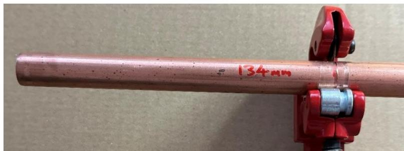
Smooth any sharp edges and clear out any copper dust from inside
